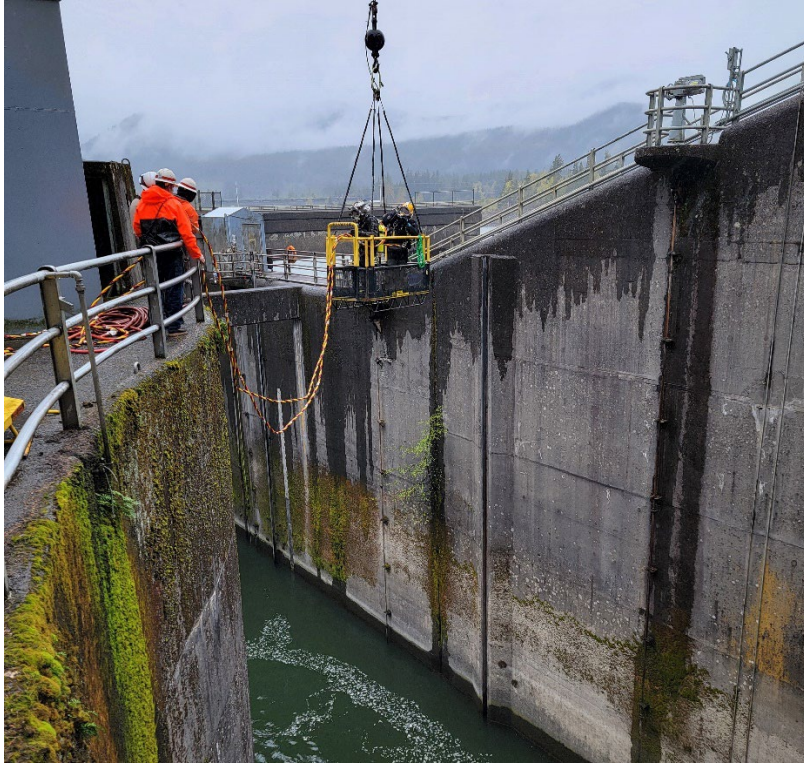
Figure 4. Divers accessing B-Branch Entrance Bay to make repairs on 04 April 2024.
